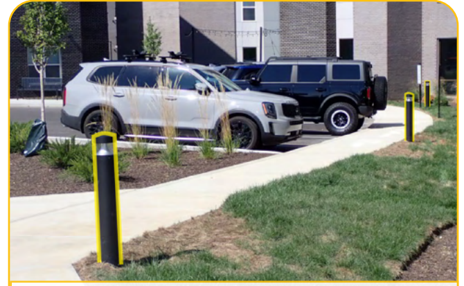
This residential development uses short, bollard-style lighting to illuminate pedestrian areas at the premise.
