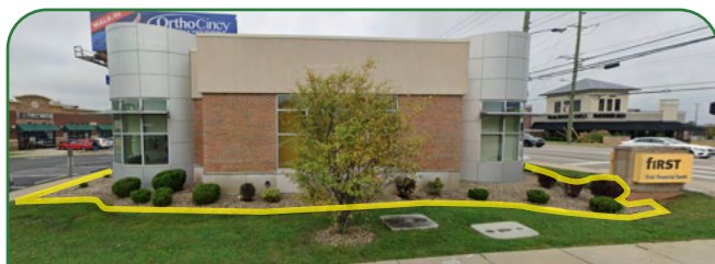
This planting bed screens the exposed building edges and foundation at this business, improving its visual appeal.
