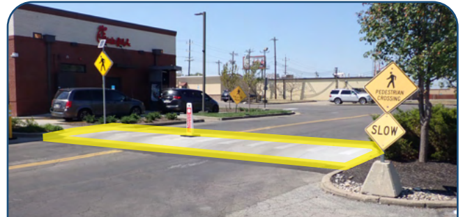
This raised crosswalk reminds drivers to watch for pedestrians who may be crossing a major driving aisle.
