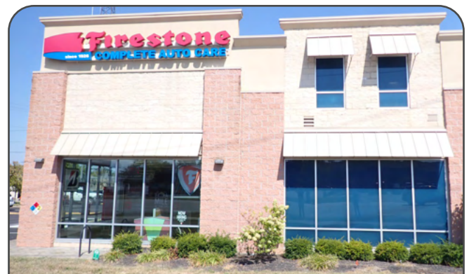
This business's facade is designed with varying heights, fake windows, and a variety of materials which provide visual interest and maintain human scale.
