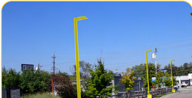
These parking lot lights are energy efficient and focus on the paved parking areas, with minimal impact to neighboring residences.
