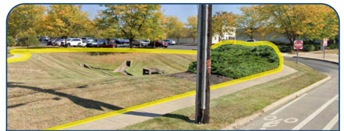
Basins or ponds should meet NPDES standards while being as attractive, integrated landscape features.
