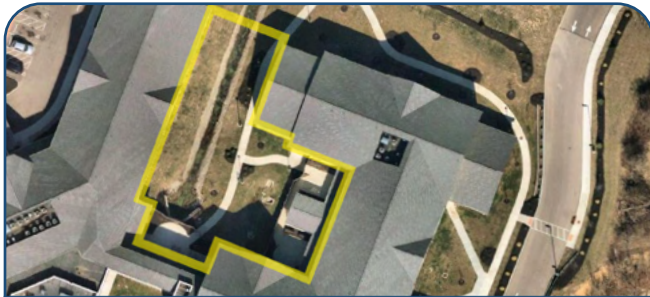
This building's use of greens, plazas, and courtyards with seating and activity areas, encourages residents to gather, walk, and enjoy the space.
