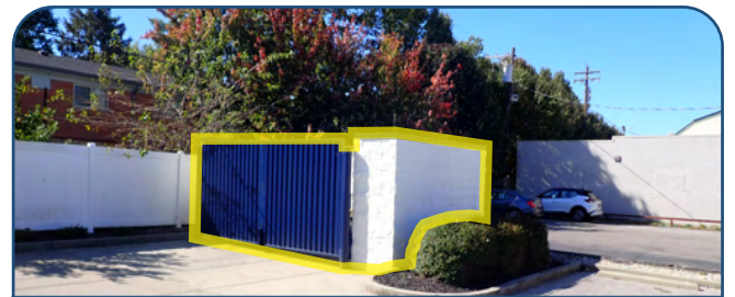
While recycling areas are encouraged, it's important to note that it needs to be screened like other services
