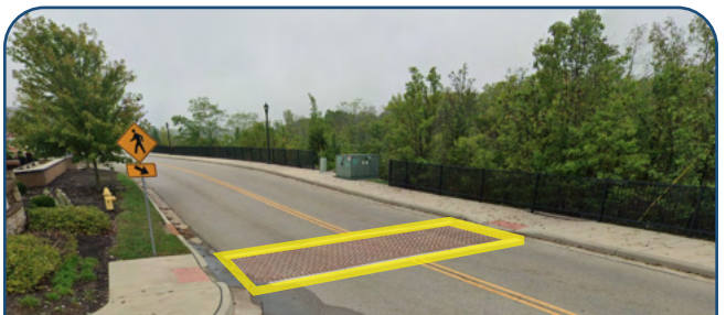
This crosswalk uses a different material from the road to match the aesthetic of the development while reminding drivers to be alert for pedestrians.
