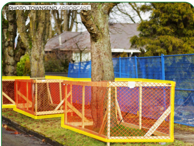
The snow fencing around these street trees will help deter any equipment from road construction from damaging the roots, protecting the overall health of these trees.
